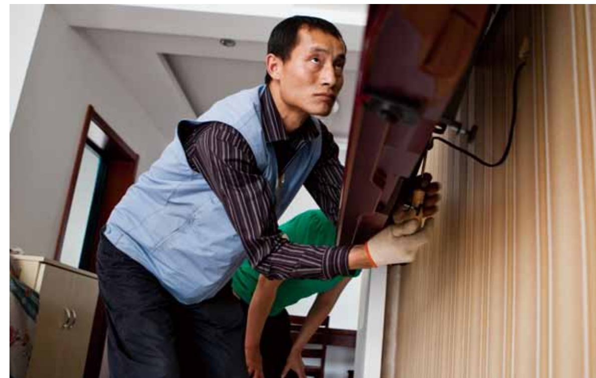
The installer tightened the TV in place.
